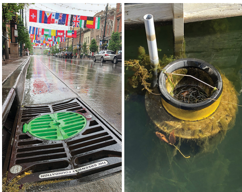
Gutter Bin (street view) and Seabin. Photos courtesy of Frog Creek Partners and WPS America
